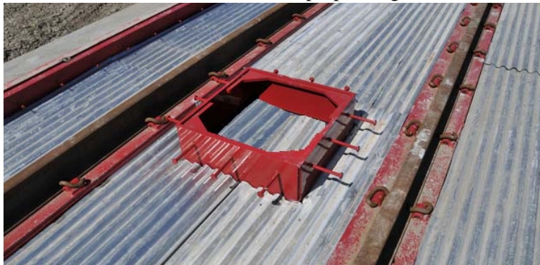
Figure 2-18. Manhole Frame
