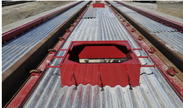
Figure 2-17. Deck Pan Installed
