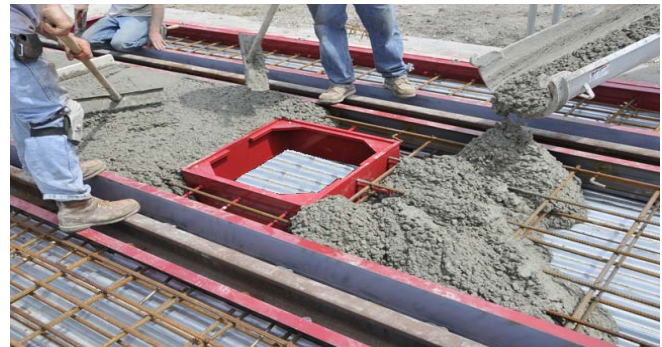
Figure 2-19. Rebar Installed (Left) and Pouring Concrete (Right)
